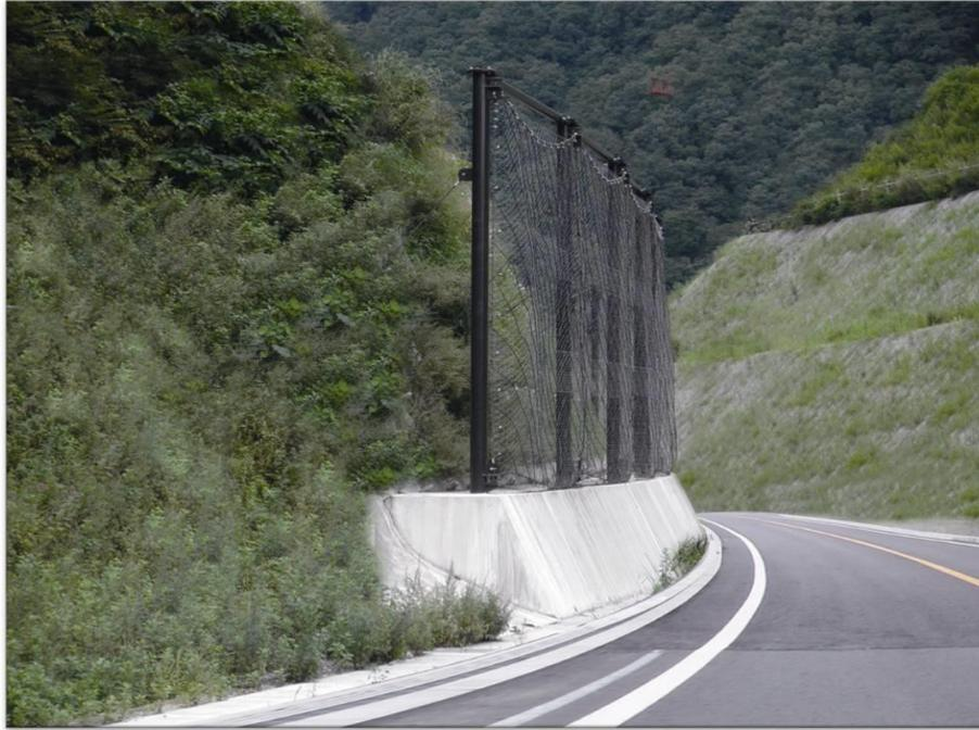
**Figure 5.1 Rockfall protection fence**
