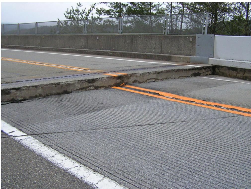
*Photo 4.1: Gap at the abutment caused by Noto Peninsula Earthquake, 2007
