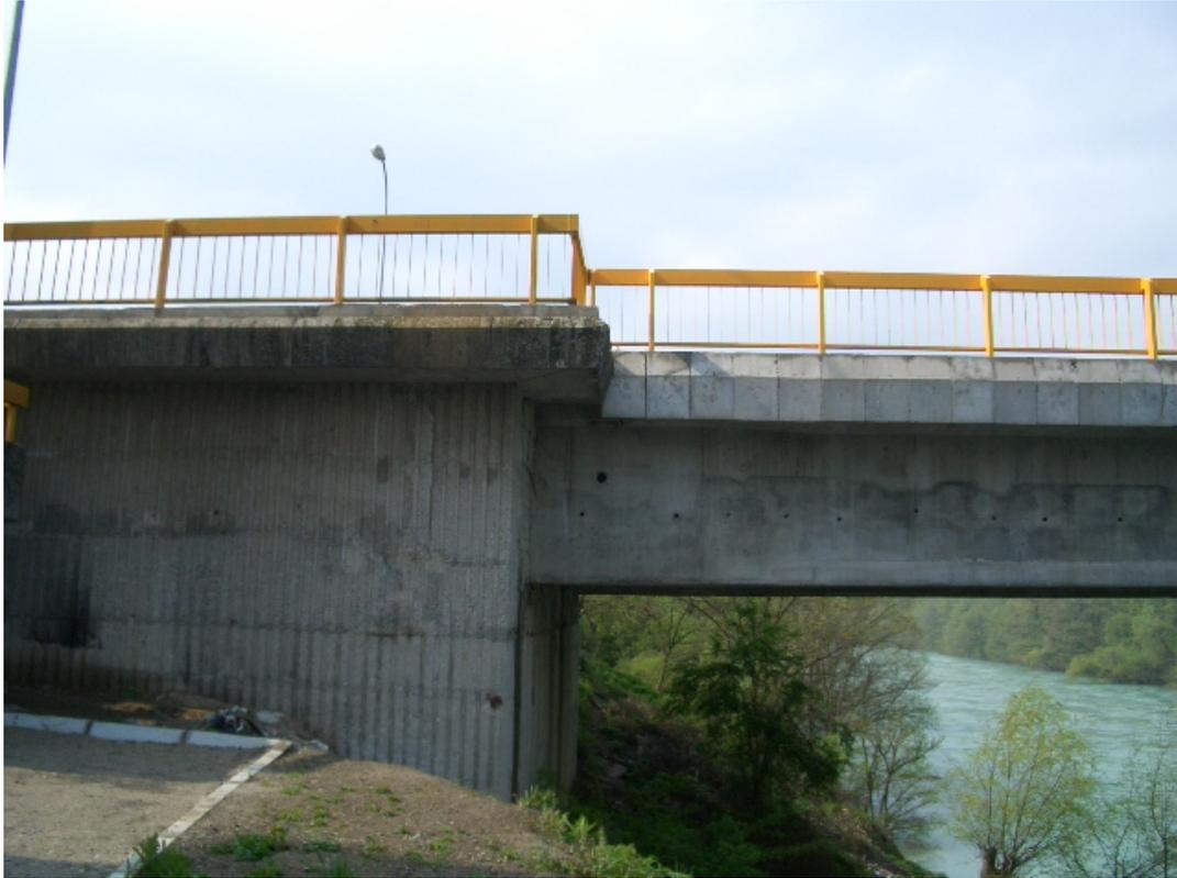
*Photo 2.8: Side view of integral abutment of Foca Bridge*
