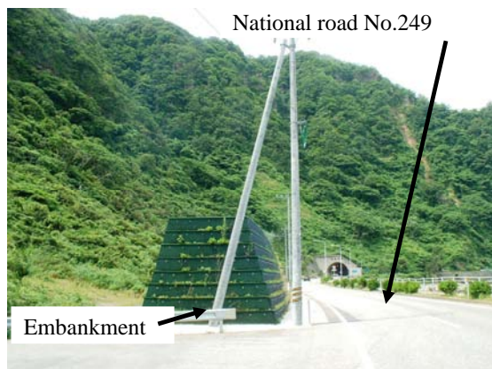
Fig. 14. Constructed embankment against rockfalls.
