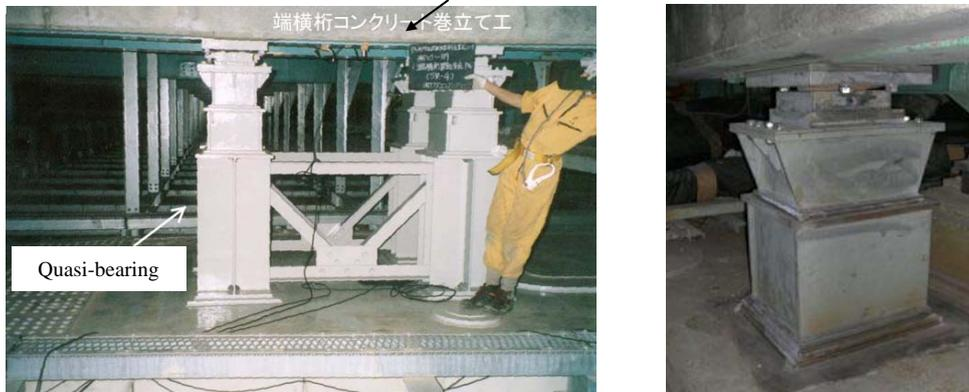
**Figure 5. Quasi-bearings and the concrete lining method of the end crossbeam**
