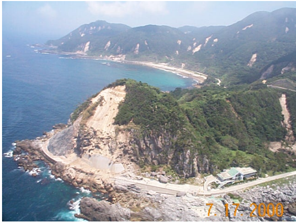
(a) Slope failure along the road from Sawajiri Bay to Nagahama Beach
