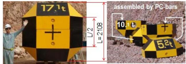
Fig. 6 RC-blocks of 17.1 ton, 10.1 ton and 5.2 ton
