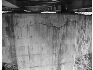
Figure 3. Large horizontal cracks in center of pillow beam.
