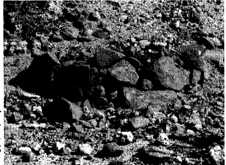
Base of north-west tower at the corner of north-west stone wall, Khorfakkan fort, looking from north-west.
