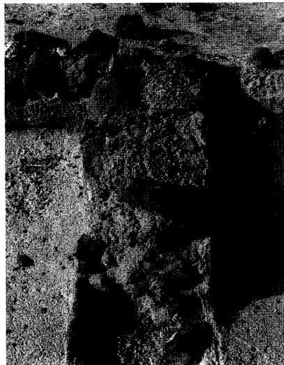
Wall of Rooms, Khorfakkan fort. Stones were piled up with pink mud mortar including small white smashed shell and white lime. Surface of walls was plastered by the same mud mortar with thickness of 2-3cm.
