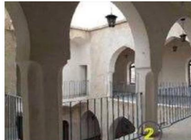
d. Most windows open to the inside.
