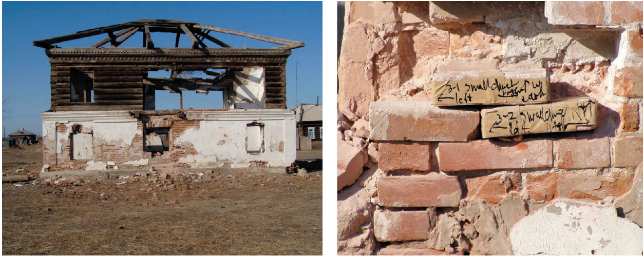
Fig. 3. In left picture: general view of location “Small church” (N 50°39’39’’; E 79°18’42’’), Dolon’ village. The first floor of the building was constructed from bricks, the second floor – from wood. The length of front wall is 14 m. Total height of the building is 6 m (from the ground level to the roof), the height of the first floor is 3 m. Mean thickness of the mortar on the wall is about 1 cm. The left side of the left window and the right side of the right window are located at the distance of 170 cm from the left and the right edges of the wall, consequently. The width of the left window is 130 cm; the width of right window is 95 cm. The height of these windows is 130 cm. The width of the central window is 150 cm; the height of the central window is 110 cm. The distance between the upper edges of the windows and the ground level is 225 cm. In right picture: location “Small church”, Dolon’ village. The bricks from the wall, which is located to the right from the central window, were selected for the sampling. The lower brick was selected for International Intercomparison (sample KSD 3-2). The distance between the left surface of KSD 3-2 brick and the right side of the central window is 33 cm. The distance between the bottom surface of KSD 3-2 brick in the wall and the ground level is 107 cm.
