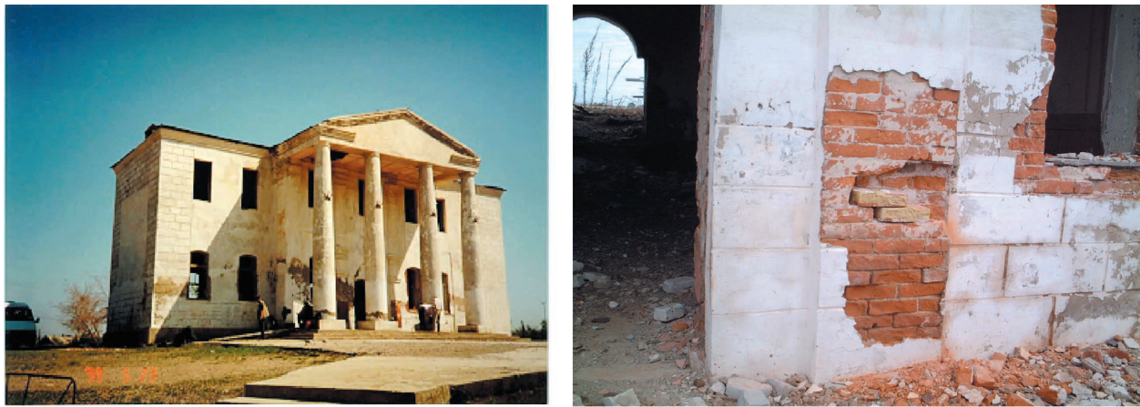
Fig. 4. In left picture: general view of location “Large church” (N 50°39’42’’; E 79°18’34’’), Dolon’ village. The detailed description of the building is presented in the reference. 4) In right picture: location “Large church”, Dolon’ village. The bricks from the wall to the right from the central entrance were selected for the sampling (sample KSD 1-3 and sample KSD 2-1 – lower brick). The portico of the building was constructed several years after the nuclear test on 29 August 1949. The distance between the left surface of KSD 1-3 brick and the right side of the central entrance is 82 cm. The distance between the left surface of KSD 2-1 brick and the right side of central entrance is 94 cm. The distance between the bottom surface of KSD 1-3 brick and the floor of the portico is 111 cm. The distance between the bottom surface of KSD 2-1 brick and the floor of the portico is 102 cm. The height of the central entrance is 3 m; the width of the central entrance is 2 m. Mean thickness of the mortar on the wall is about 1.5 cm.
