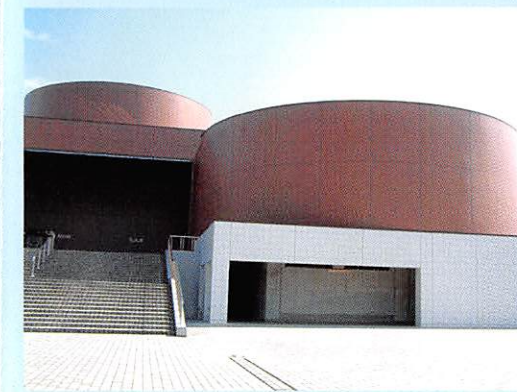
外観 External Appearance
