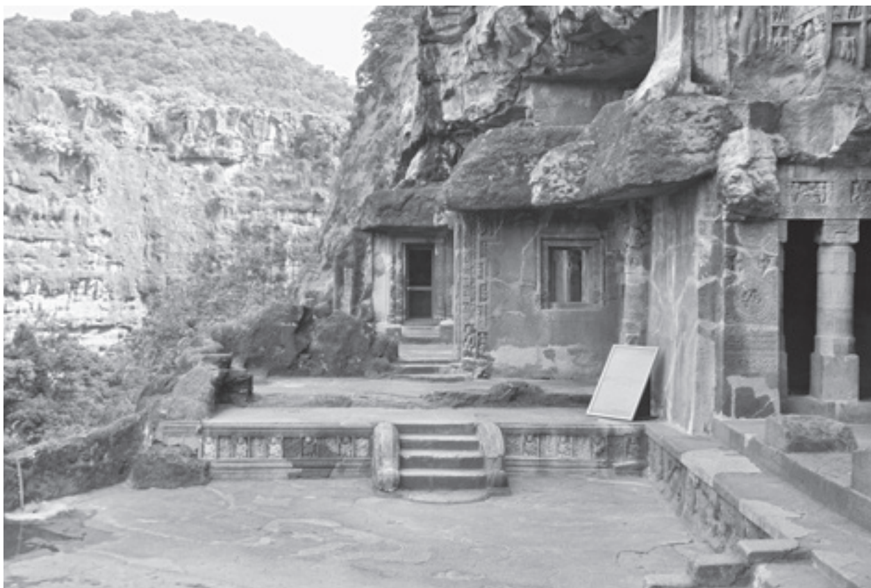
Fig.146 Ajanta Cave 26LW Façade
