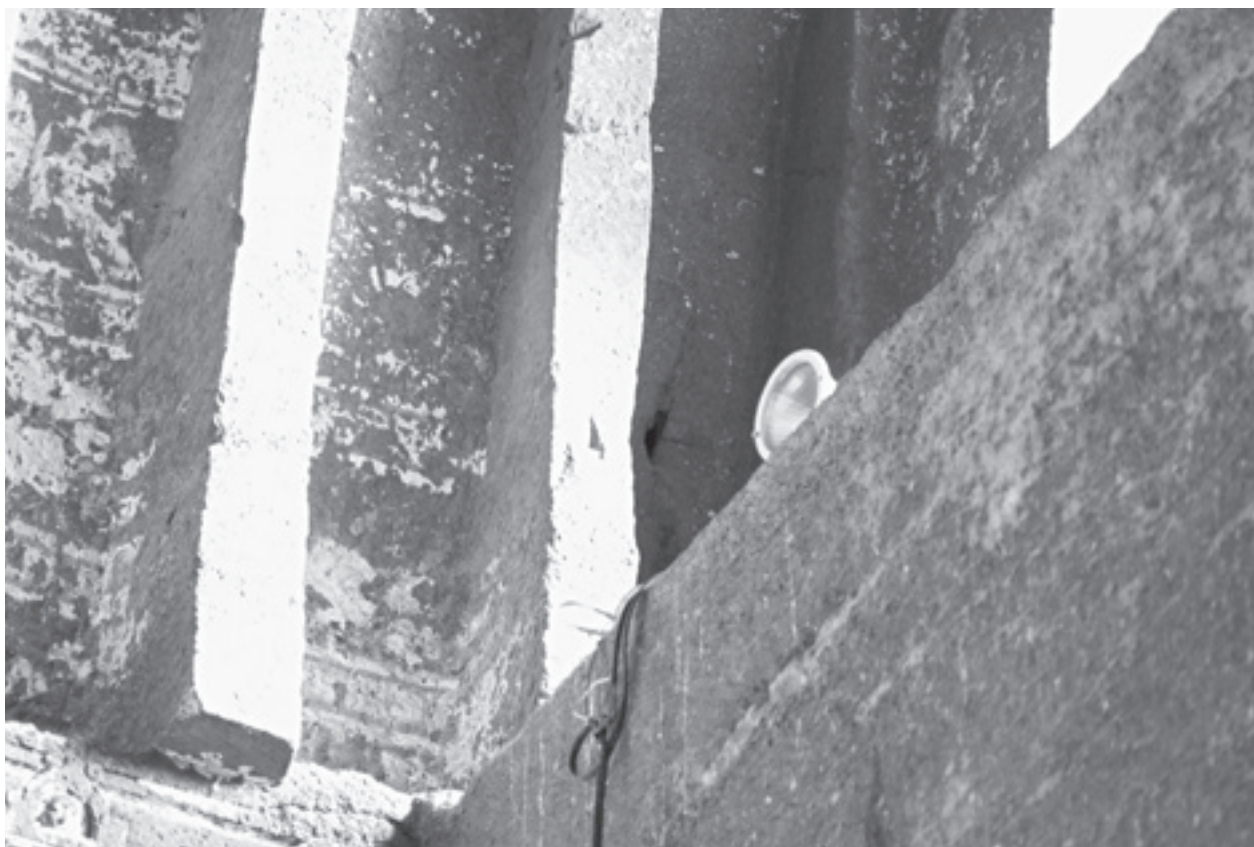
Fig.142 Ajanta Cave 26 Interior, Ceiling
