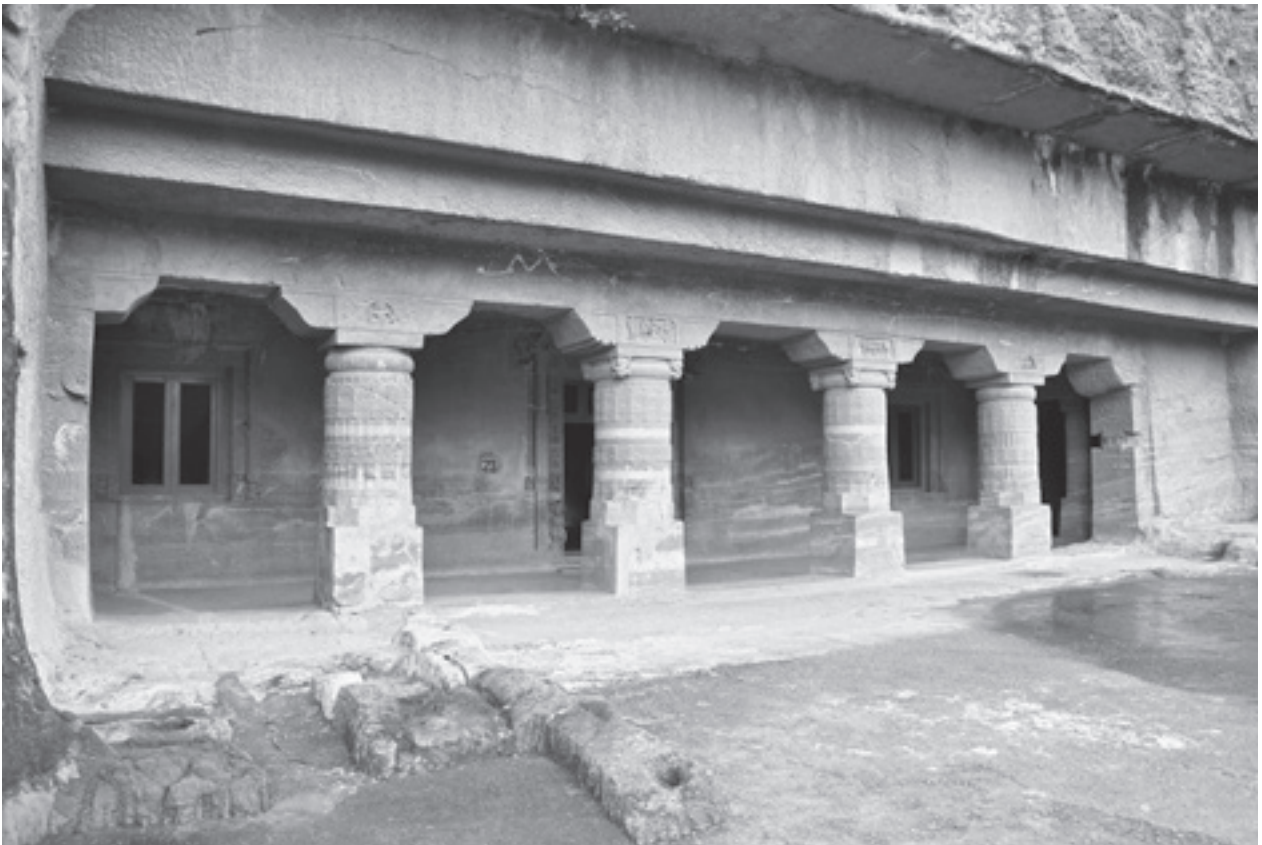
Fig.108 Ajanta Cave 23 Facade
