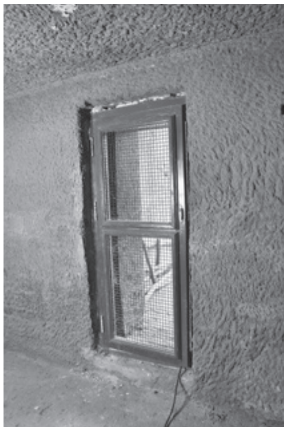
Fig.150 Ajanta Cave 27 Porch Cell, Interior
