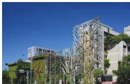
Figure 6. A completed work of the Green Gate
