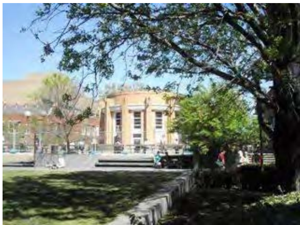
Frank Tate Building 外観
