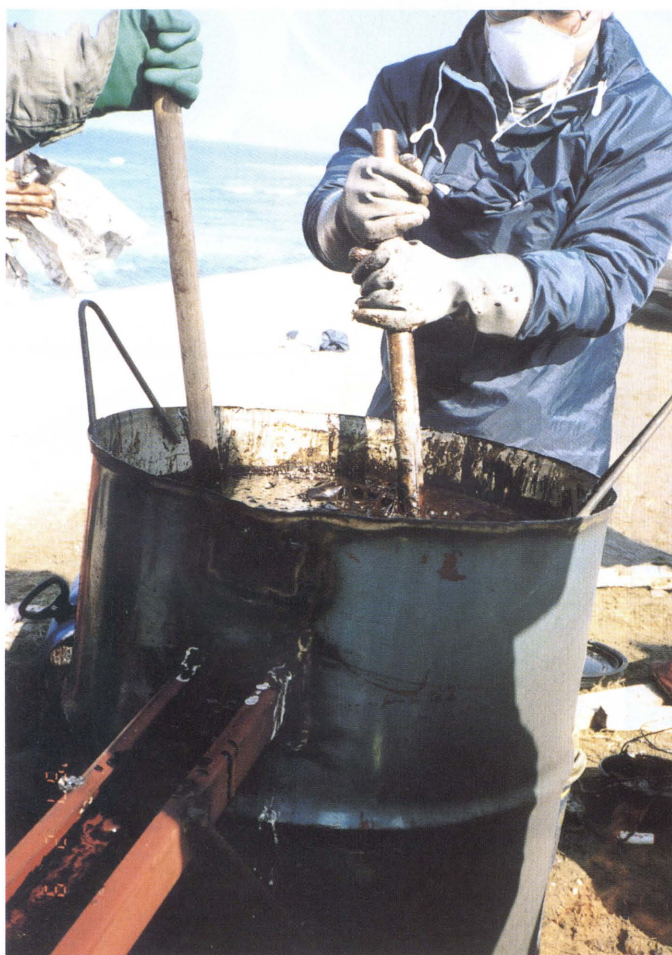
Figure 19 Separation tasks of heavy oil and sands or gravels on the site. Warming up seawater in about 40 °C , adding contaminated sands or gravels, then getting the oil on the surface.
