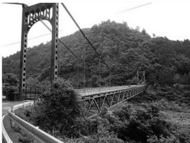
Fig. 1-1 Bridge in Hamamatsu city which was made in 1956 collapsed in the heavy rain of 2015 (1) .
