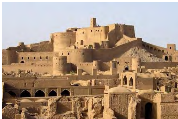
Photo 1.4 Arg-e bam in Iran was destroyed in 26th December 2003.
