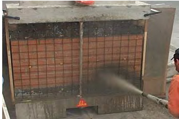
Photo 3.5. Applying Shotcrete on a masonry wall.
