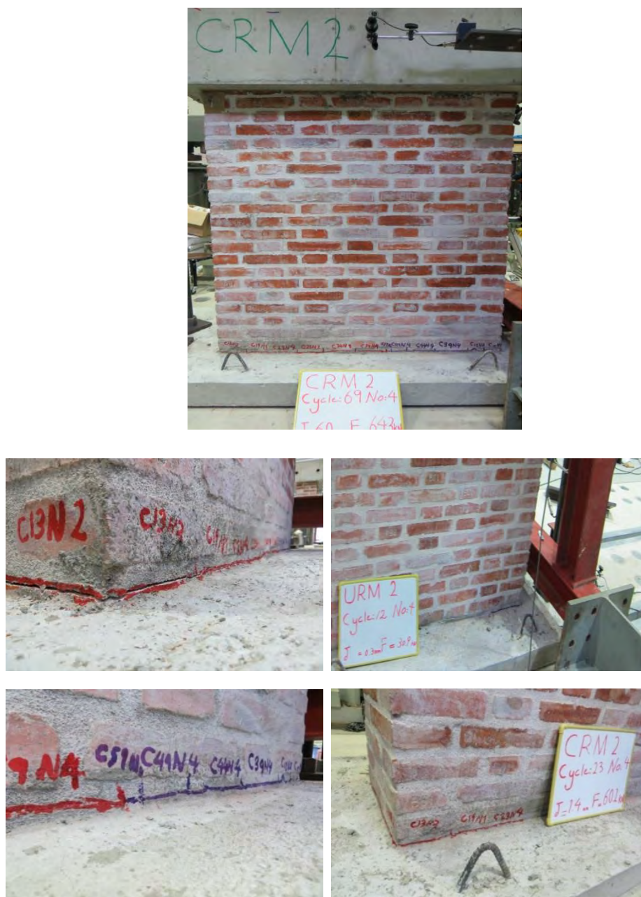
Photo 4.12. Cracking pattern and failure modes of the specimens.
