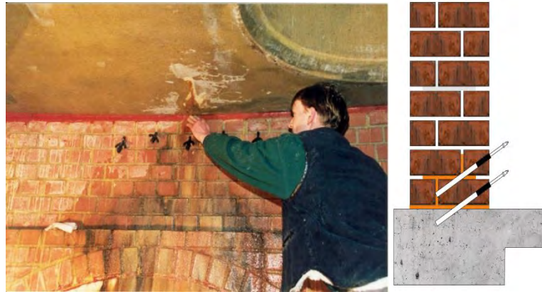
Photo3.8. Applying injection method for existing masonry brick wall.
