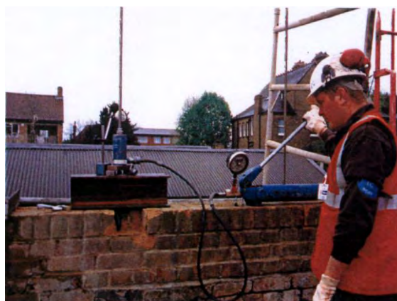
Photo 3.7. Applying Post-tensioning method.
