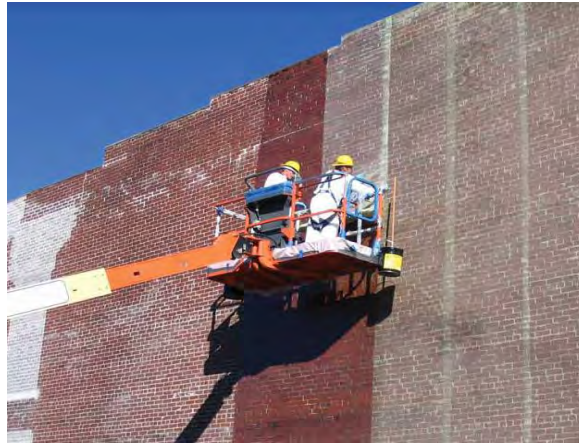
Photo 3.6. FRP retrofitting method.
