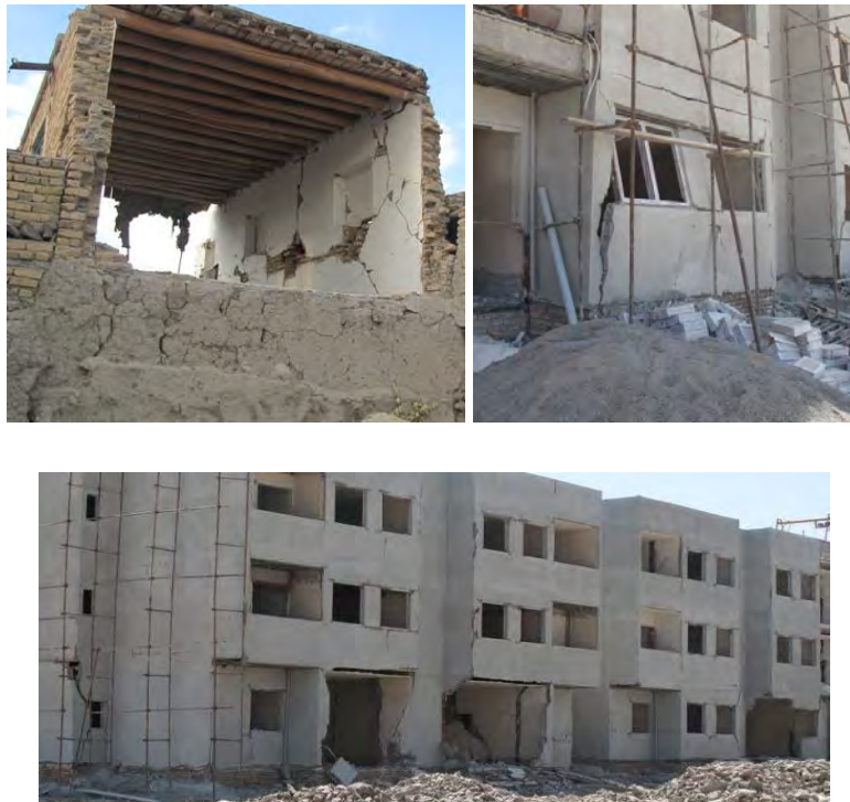
Photo 3.3 Out of plane behavior of masonry walls in case of seismic orthogonal loads.
