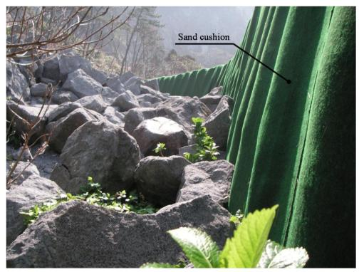
Figure 3.1 Rockfall protection wall with a sand cushion
