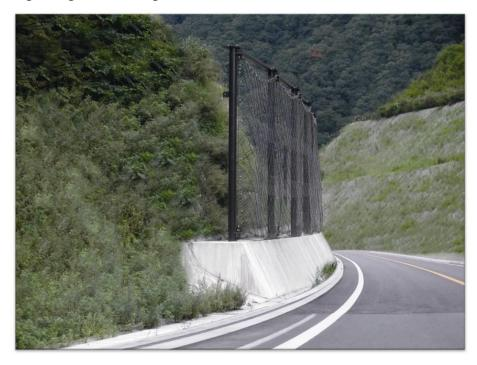
Figure 5.1 Rockfall protection fence
