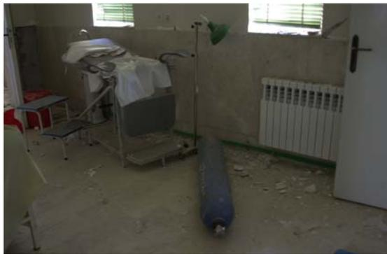
Photo II.1- Falling over of a gas cylinder
