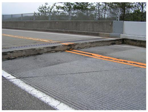
Photo 4.1: Gap at the abutment caused by Noto Peninsula Earthquake, 2007 (By favour of Hiroshi MASUYA)
