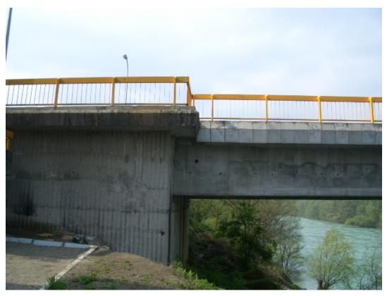
Photo 2.8: Side view of integral abutment of Foca Bridge
