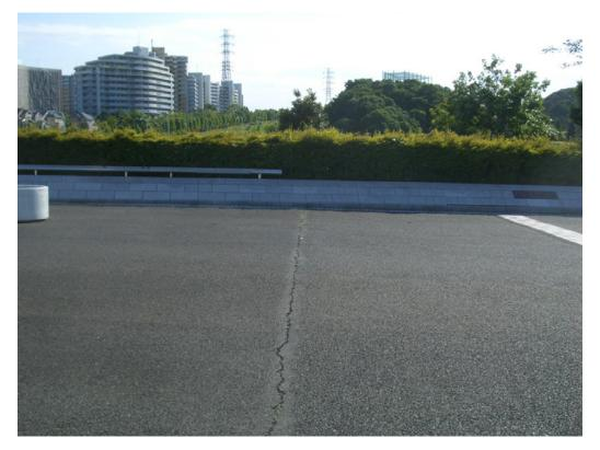
Photo 2.2: Crack of pavement at the end of approach slab of Kujira Bridge
