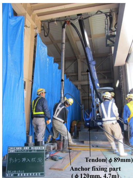
During the insertion of the anchor
