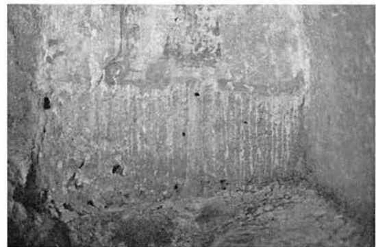
Fig.1 Lines of flowing lime paste beneath a mural painting
