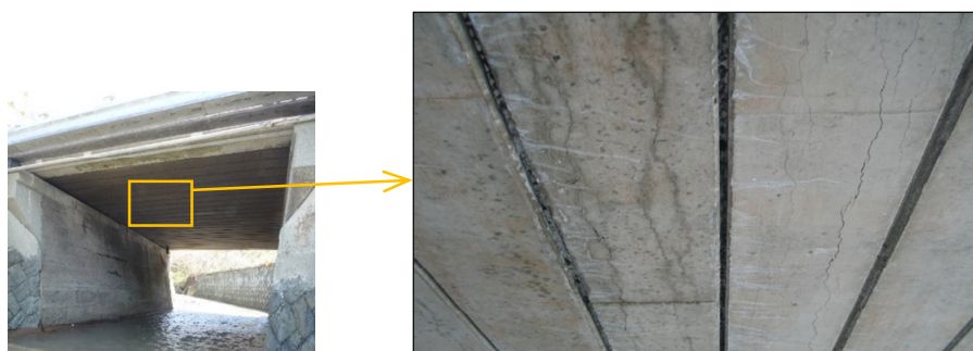
Fig. 1 Cracks occurs along with the PC strands (bottom surfaces).
