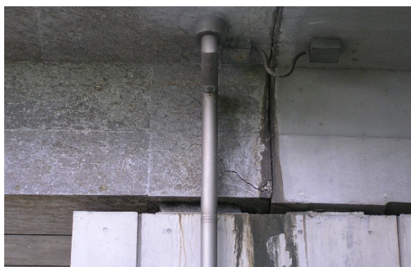
Fig. 25 Cracks occurred at the end of PC girder due to ASR-induced deformation.
