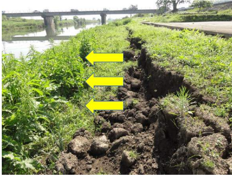
Figure A.17 The lateral spreading occurred at Kiyama Riverbank, Akitsu town
