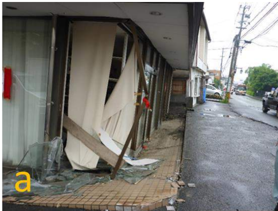
Figure 2.12 Damaged buildings caused by liquefaction-induced ground deformation
