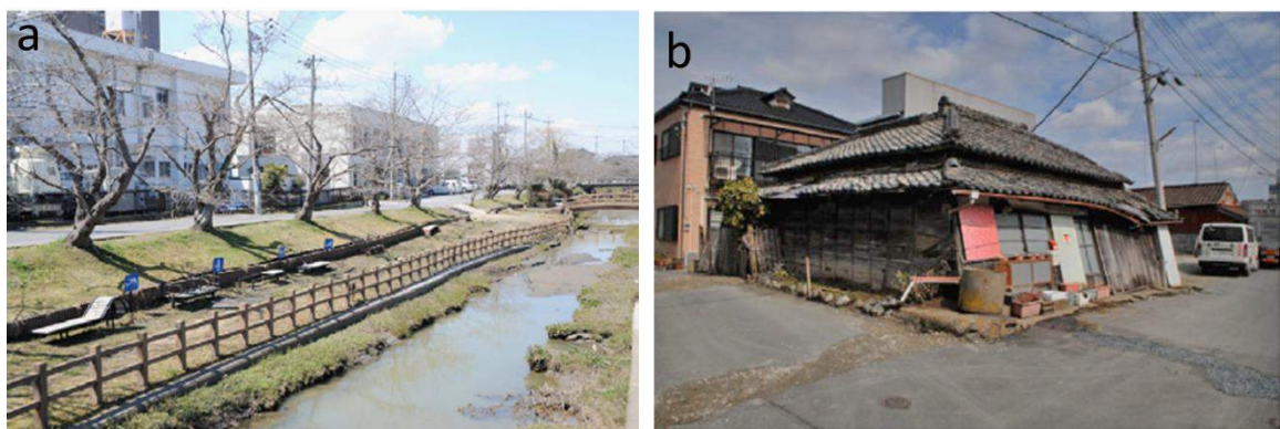
Figure 2.7 Liquefaction-induced lateral spreading in the 2011 Great East Japan earthquake (a) Lateral ground spreading towards the river (b) Damaged house caused by lateral spreading
