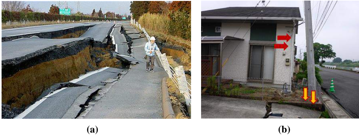
Figure 1.1 Liquefaction-induced damages: (a) The damaged road in the 2011 Great East Japan earthquake (b) Tilted residential house in the 2016 Kumamoto earthquake
