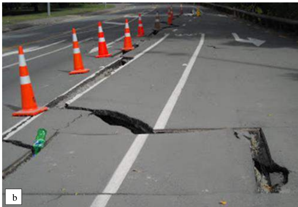
Figure 3.2 the lateral spreading due to liquefaction during the 2010-2011 Canterbury earthquakes
