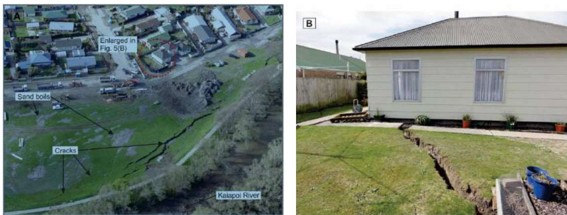
Figure 2.9 Lateral spreading occurred in the 2010-2011 Canterbury earthquakes, New Zealand
