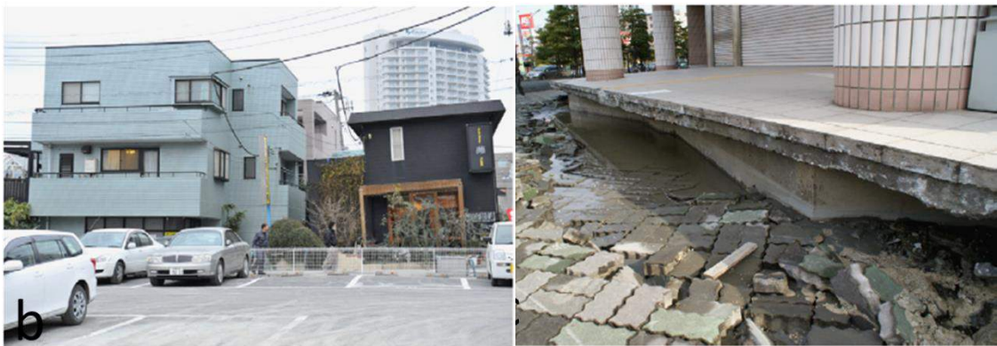
Figure 2.6 Damages caused by liquefaction in the 2011 Great East Japan earthquake: (a) A large settlement of the building (b) Tilted building (c) Ground settlement around the pile-supported building
