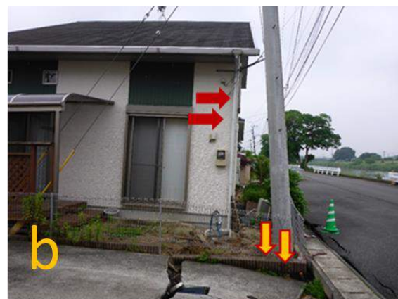
Figure 2.12 Damaged buildings caused by liquefaction-induced ground deformation
