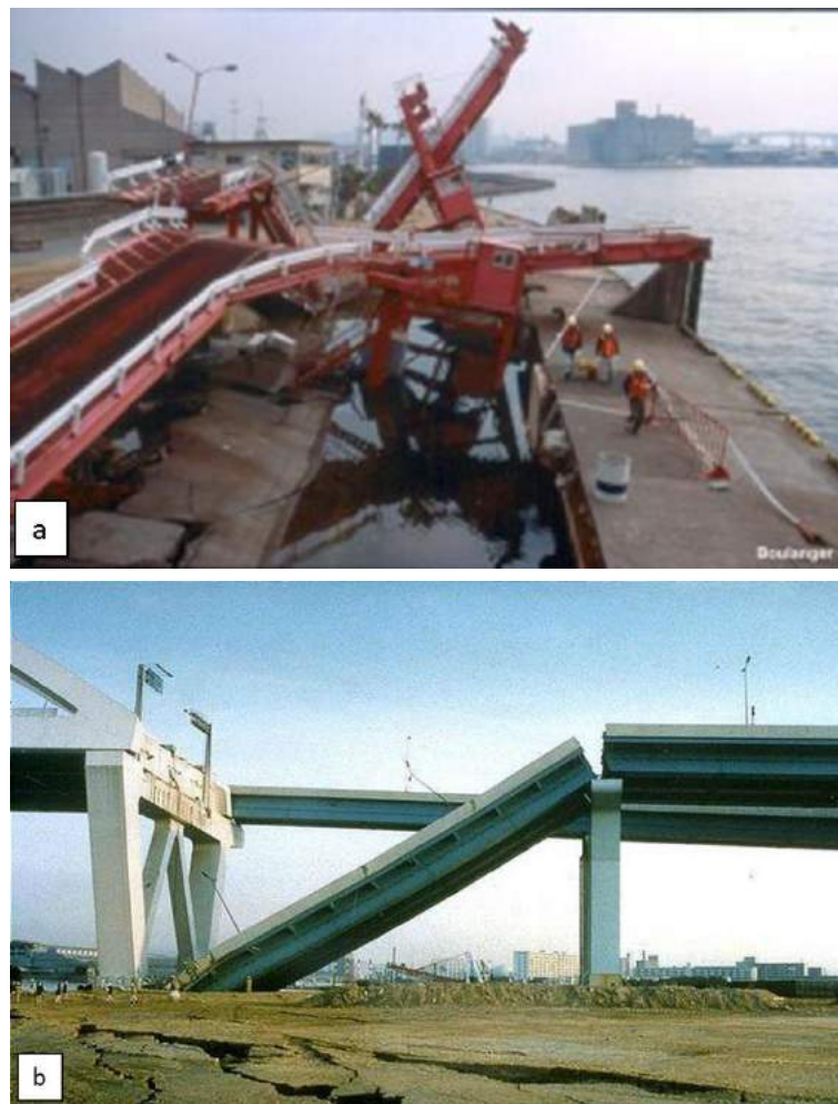
Figure 3.1 The lateral spreading due to liquefaction during the 1995 Kobe earthquake (a) The collapsed ferry terminal (b) The collapsed Nishinomiya bridge
