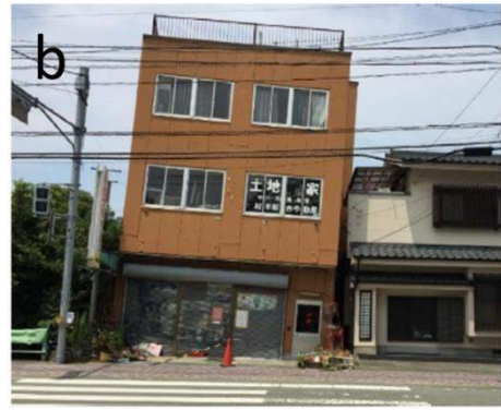
Figure 2.11 Buildings suffered from differential settlements due to liquefaction
