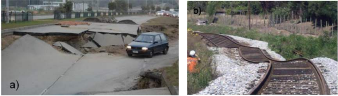
Figure 2.1 Post-liquefaction settlements in the 2010 Chile earthquake: (a) Costanera route in Concepcion City (b) Near Concepcion City
