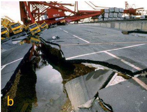
Figure 4.1 Damaged constructions due to liquefaction-induced ground displacements;
