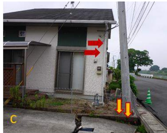
Figure 4.1 Damaged constructions due to liquefaction-induced ground displacements;
