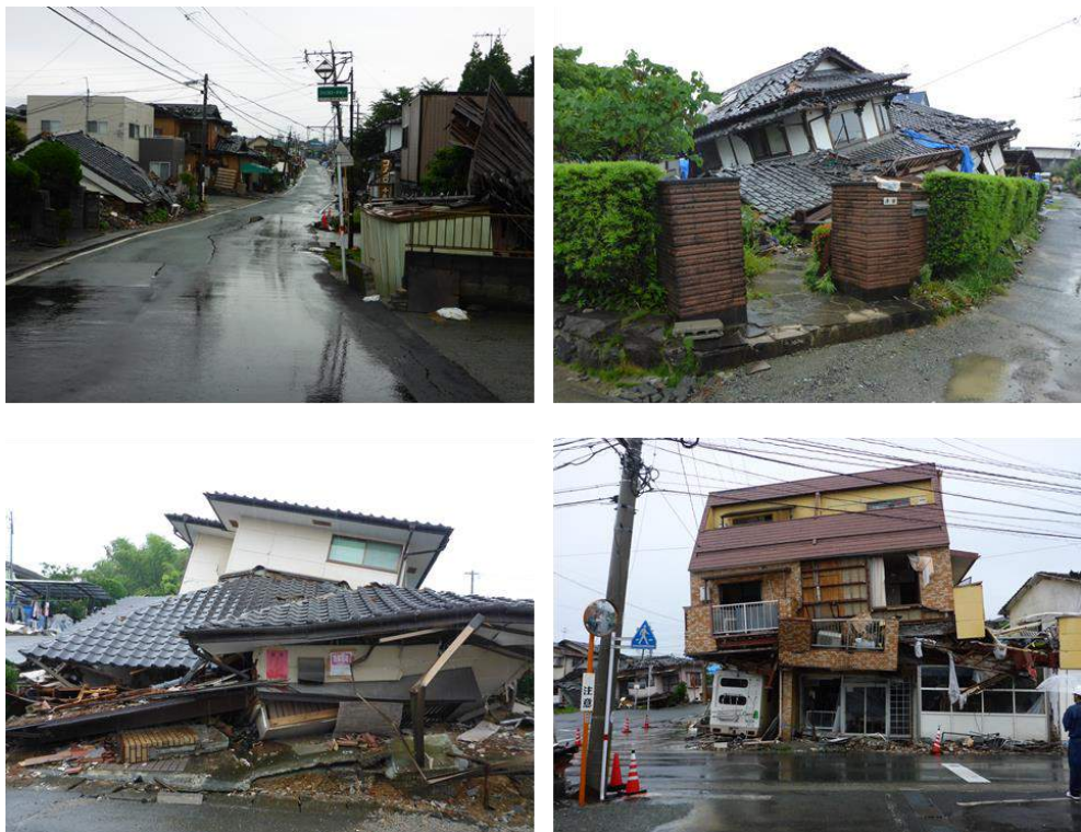
Figure A.4 The residential houses damage in Mashiki town
