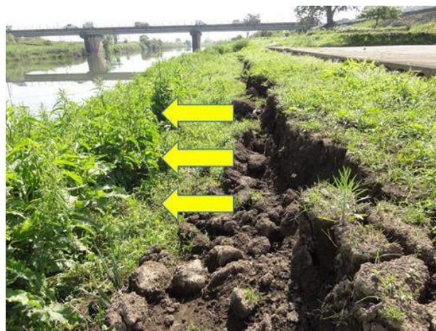
Figure 2.13 Lateral spreading in the river bank of Kiyama River, Akitsu Town, Kumamoto
