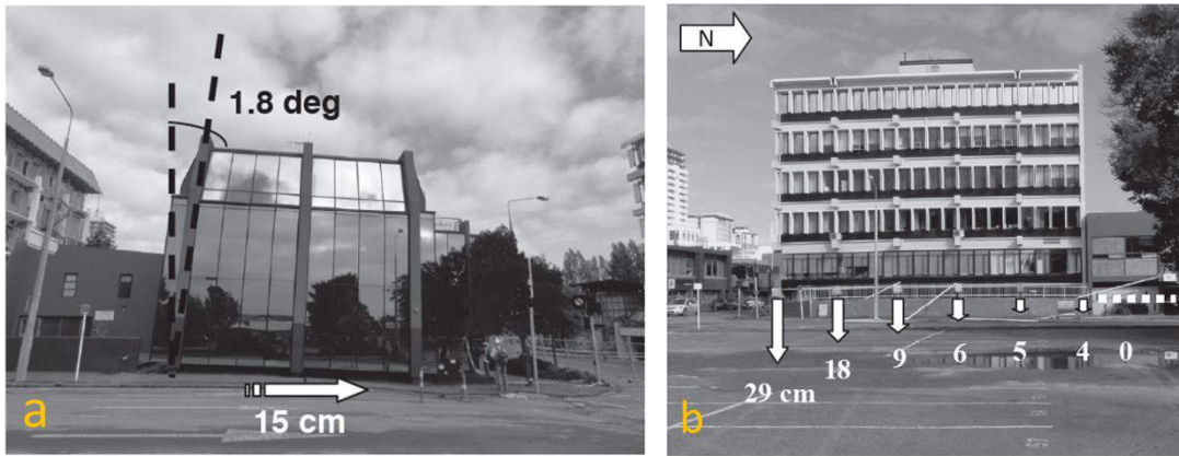
Figure 2.8 Tilted buildings due to liquefaction-induced differential settlements
