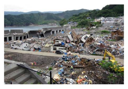
Figure 1. Damage to A Large Embankment (Photo by Ryohei Yamashita on June 2011)
