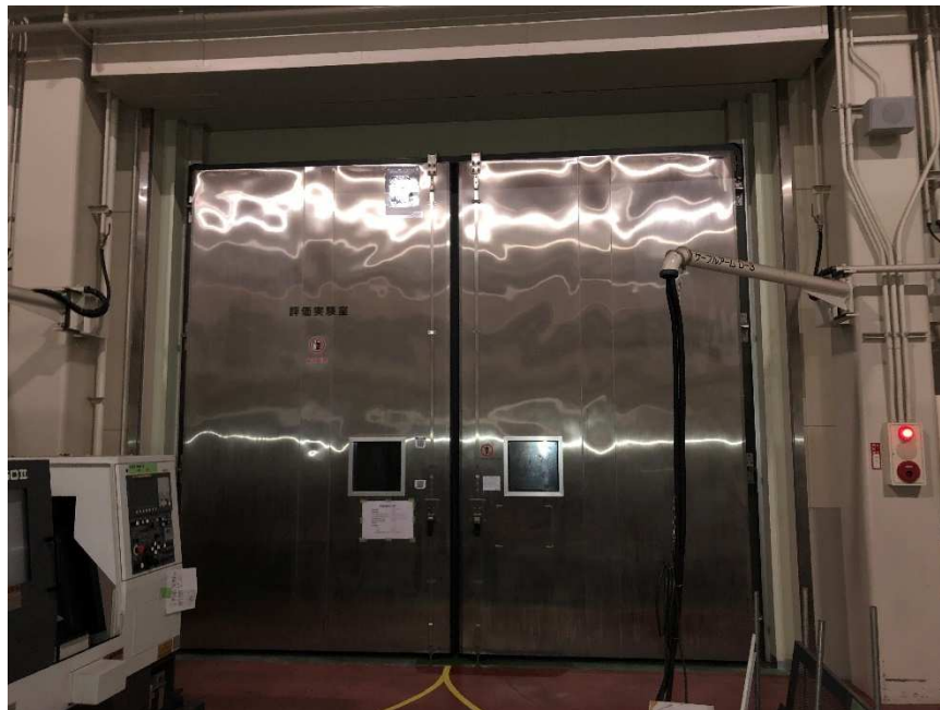
Fig. 6-3 Environmental testing laboratory (Exit door side)
