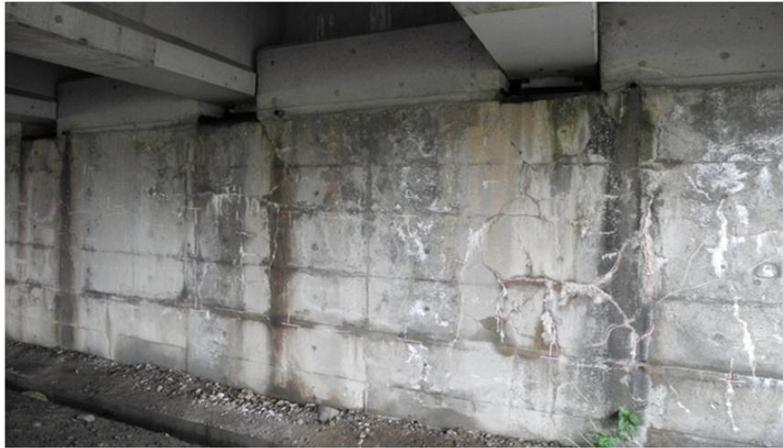
**Figure 2.1** Abutment A deteriorated by ASR
