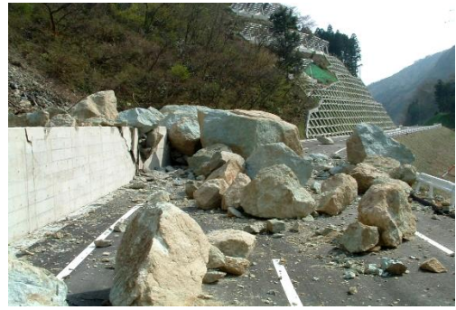
b) Disaster of new road by rockfall
