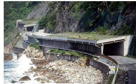
d) Rock shed
