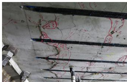
Figure 2.1 Reinforced bridge deck by FRP bars
