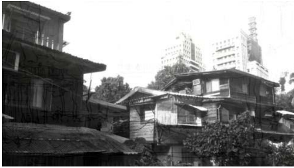
Figure 12. An informal settlement, the Shaoxing Community, in an urban renewal project shown in the performance propaganda video of the “Zhongzheng Wanhua Reviving Plan” 17
