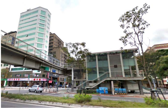
Figure 14. The pedestrian bridge crossing, Zhonghua Road.
