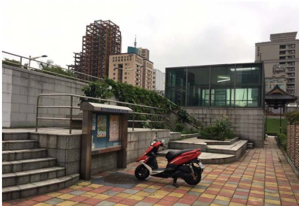
Figure 16. The emergency exits of the underground railway on Zhonghua Road
