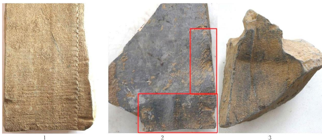
Figure 57 The fabric impressions on the concave surface of the roof tiles (Source: Photos by the author)
