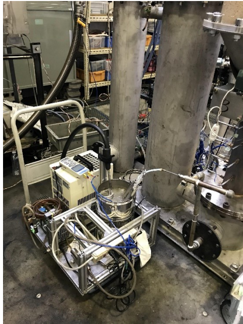
Figure 32. Real Tar Sampling Equipment Setting in The Gasifier Port
