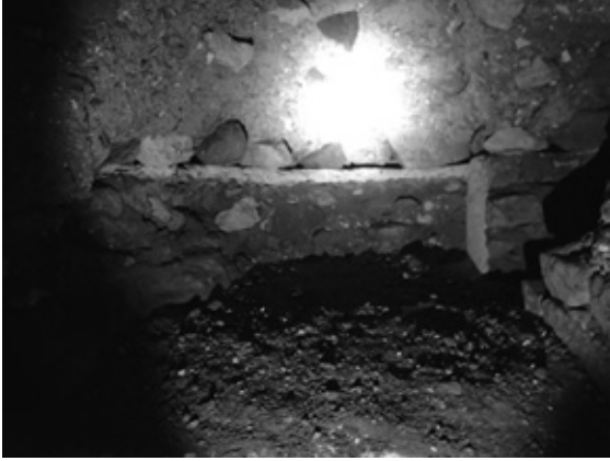
Photograph 3. Tunnel underneath Temple 11 without consolidation, possibly traces of collapse.
