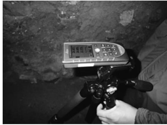
Photograph 6. Preliminary survey in the collapsed sector of tunnel I-27 in September 2017.
