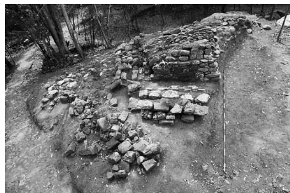
Photo 49: Two front walls from different construction stages after the excavation. The first wall has slid towards the front (Photo by Hiroyuki Ikarashi)
