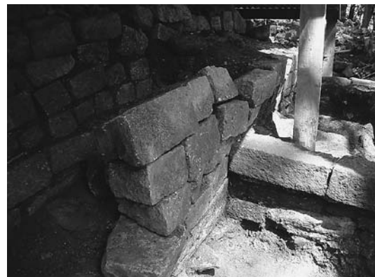
Photo 14: East buttress wall and the la trimmings of the chamber annexed on the east (both from Stage I)
