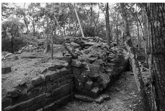
Photo 5: Butters wall in the north side of Structure 9L-101-1 st (Photo: Hiroyuki Ikarashi)
