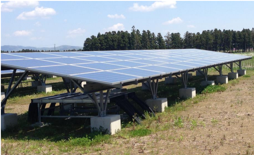
Figure 1. Large SP installed on farmland
