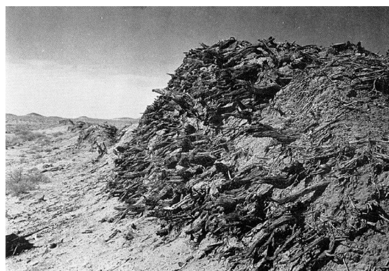
Fig. 4 XiXia long wall in Mongolia (section build of saxaul) (photo by T. Baasan in 1970s)
