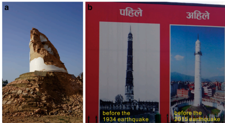
Fig. 5 The collapse of Dharahara tower. a damaged Dharahara tower; and (b) a poster showing two photos of the tower before the 1934 and 2015 earthquakes
