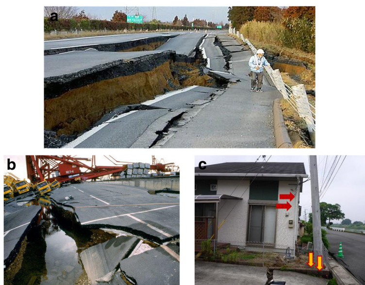
Fig. 1 a Damaged road due to liquefaction in the Great East Japan earthquake. b Damaged road due to liquefaction in the Great Hanshin earthquake, Japan. c Tilted house due to liquefaction in the 2016 Kumamoto earthquake, Japan
