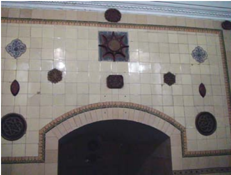
Fig-49 Demak Mosque Mihrab
