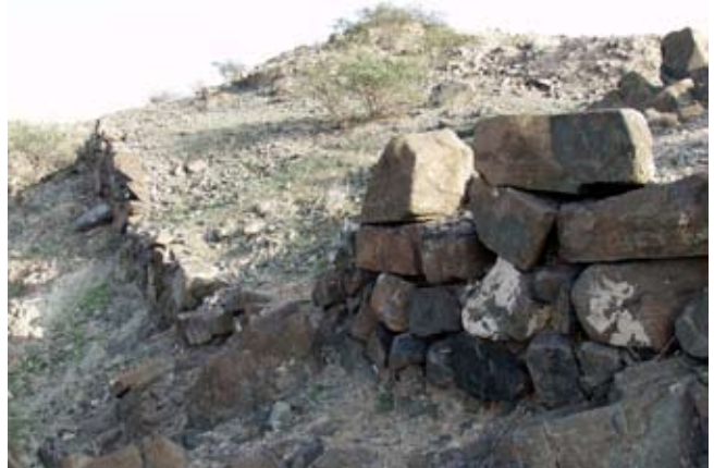
Enclosure stone wall, east side of Khor Fakkan Fort.
