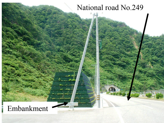
Fig. 14. Constructed embankment against rockfalls.
