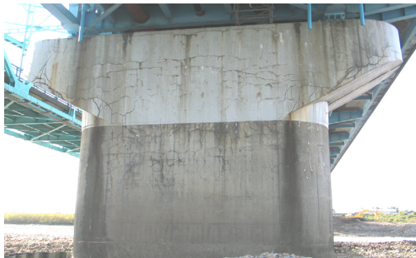
Fig. 5 Reconstruction for severely damaged ASR-deteriorated bridge pier.
