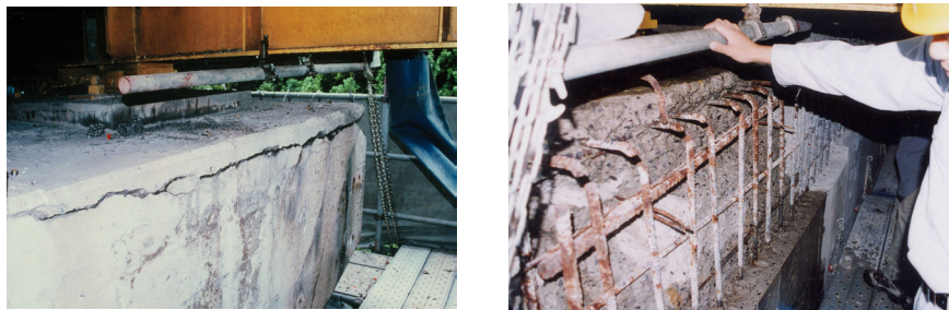
Fig. 4 Fracture of steel reinforcing bars in ASR-deteriorated bridge pier.
