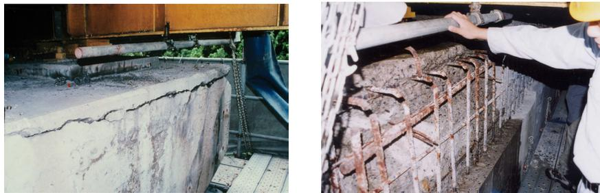
Fig. 4 Fracture of steel reinforcing bars in ASR-deteriorated bridge pier.
