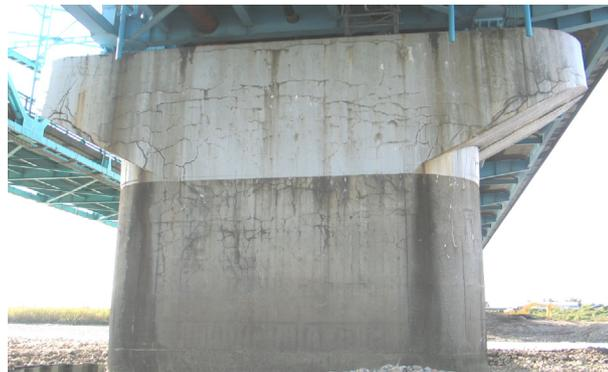
Fig. 5 Reconstruction for severely damaged ASR-deteriorated bridge pier.
