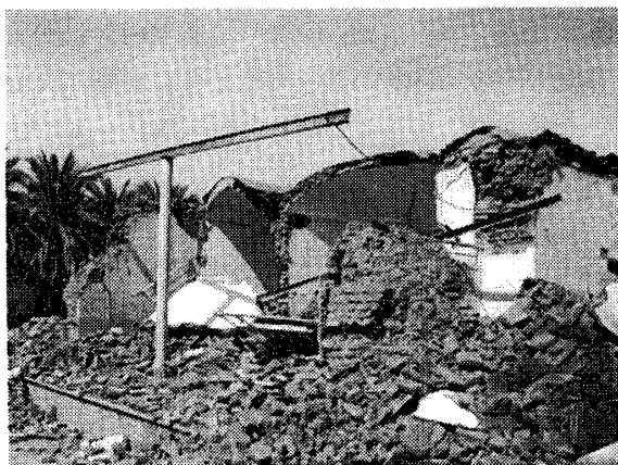
Photo 8 Damaged residential housing made of adobe bricks
