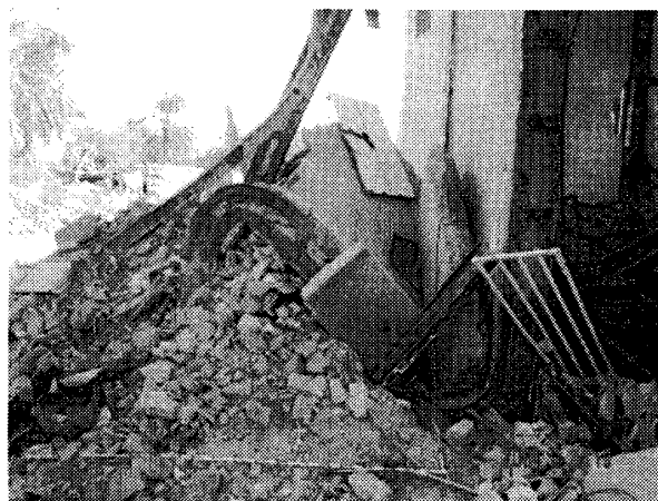
Photo 13 Collapsed steel frame building near by the water tank. This building was dislocated about 1.3 meters westward (rightward)
